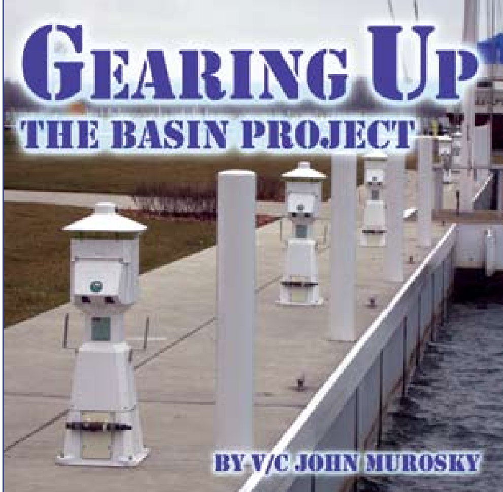
The same electric and water pedestals as used in front of the Club will be installed along the north wall when this portion of the overall basin initiative is completed this spring.
