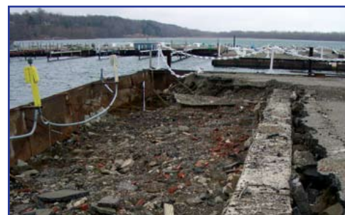
The north wall under construction with excavation and the new "deadman" in place.
